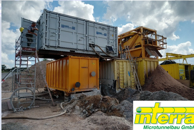
➤ GHT 390_ Baustelle Furth/ Erlangen 2017 (interra)
